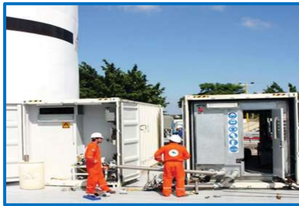
ATC & NME Tank Cleaning Modules being Set-Up at Tank Cleaning Site.
