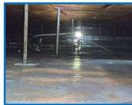
ATC NME WELL-CLEANED TANK
