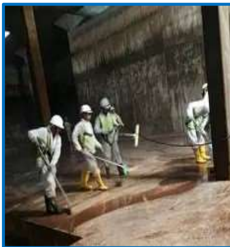
FINAL TANK MOP-UP CREW AT WORK
