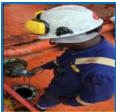
TANK ATMOSPHERE MONITORING
