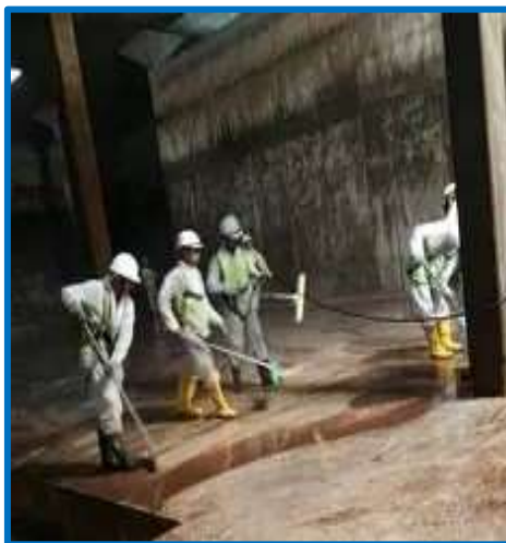
FINAL TANK MOP-UP CREW AT WORK
