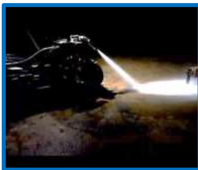
REMOTE-OPERATED JETS IN TANK
