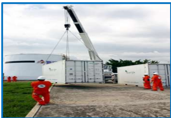
SWDA's ATC & NME Tank Cleaning 4 Modules Mobilised to Tank Site in Ireland.
