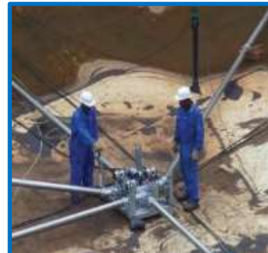
ARRAY 8 - 16 SPRAY NOZZLES
