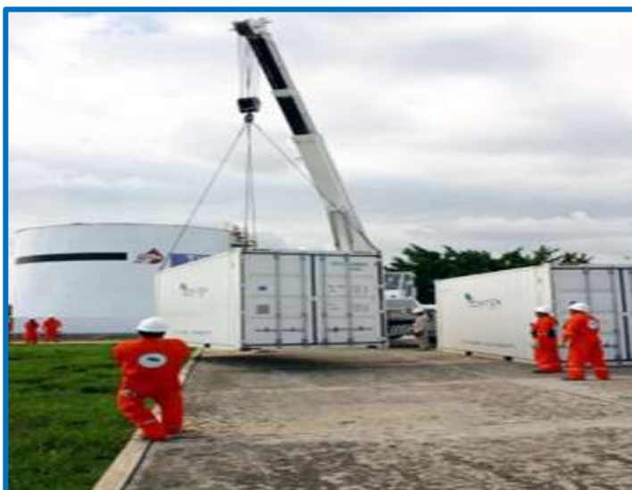
SWDA’s ATC NME Tank Cleaning 4 Modules Mobilized to Tank Site in Ireland.
