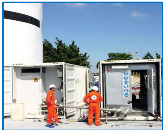
ATC NME Tank Cleaning Modules being Set-Up at Tank Cleaning Site.
